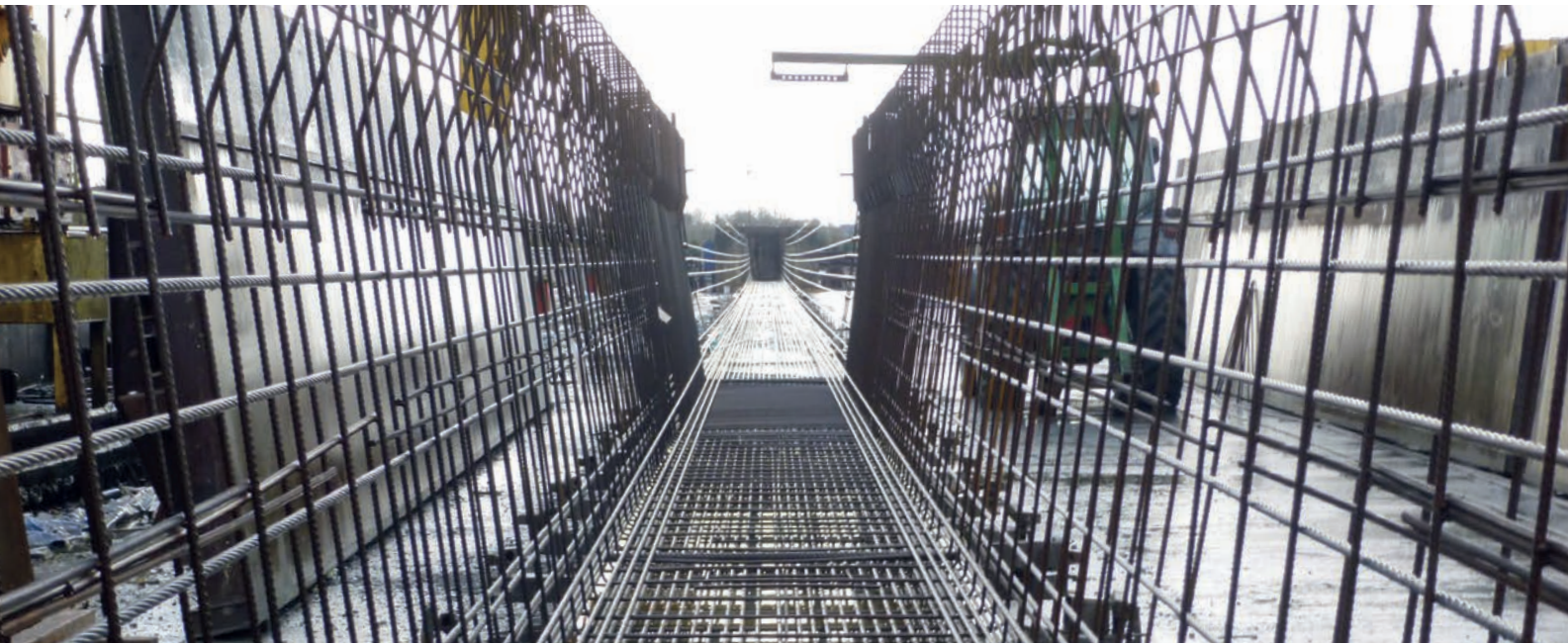
Figure 4 Pre-tensioning bed (Banagher Precast Concrete)
