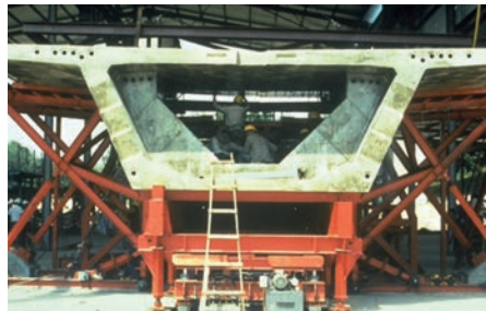
Figure 8 Internal cable ducts at pier (STAR LRTS Viaducts, Malaysia)
