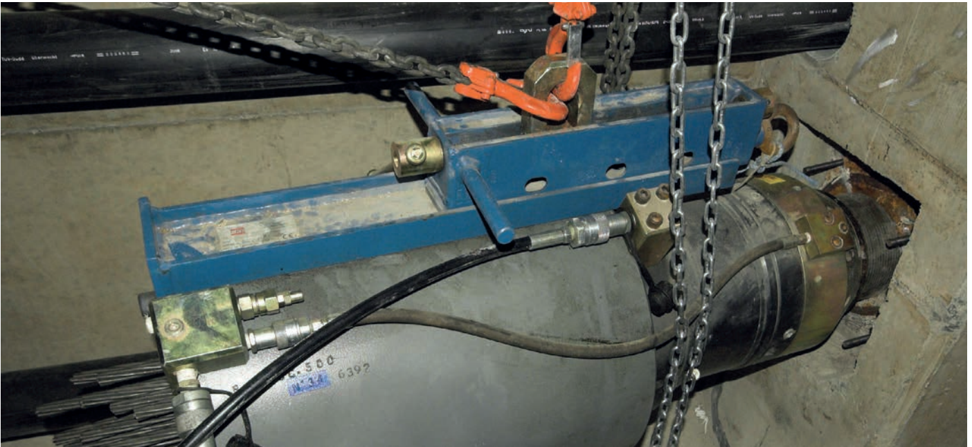
Figure 6 Post-tensioning jack stressing a cable (Clackmannanshire Bridge, UK)
