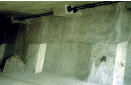
Figure 7 Anchorage blisters inside box (East Moors Viaduct, UK)
