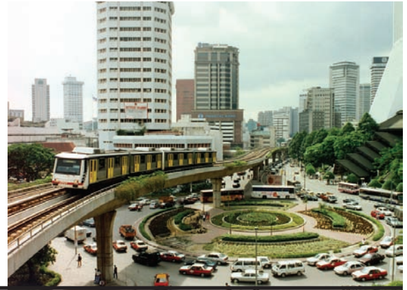
→ Figure 3 STAR LRTS Viaducts, Kuala Lumpur: 35m spans over land
