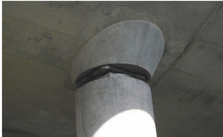
Figure 7 Pinned bearing: Broadmeadow Estuary Bridge
