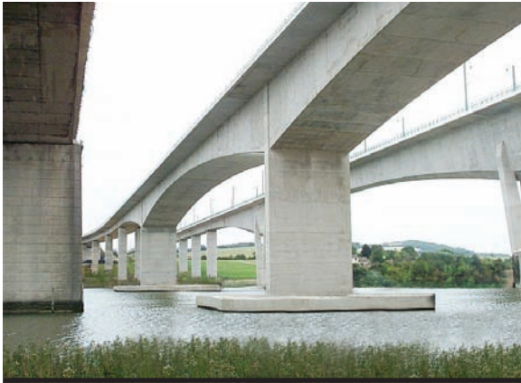
← Figure 2 Medway Crossing Viaducts: 152m spans over deep water
