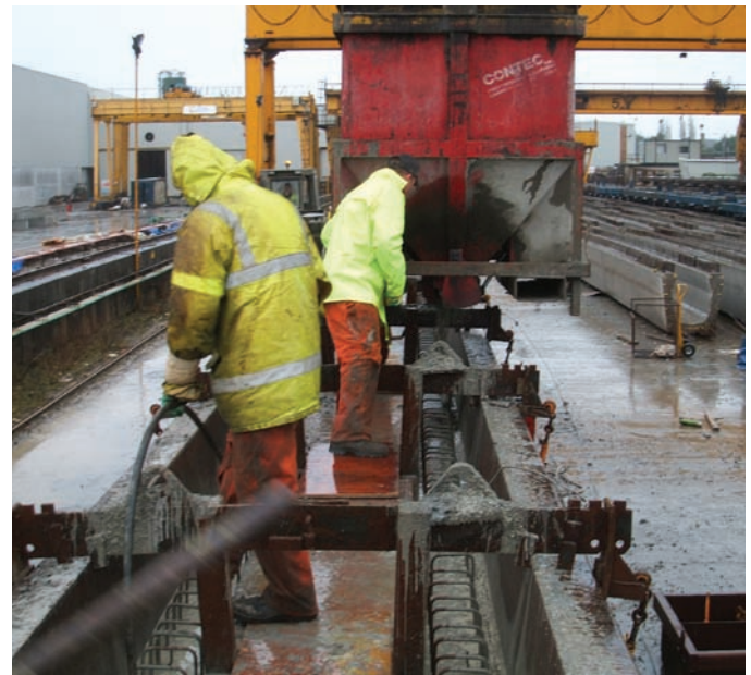
Figure 5 Casting a concrete beam (Banagher Precast Concrete)
