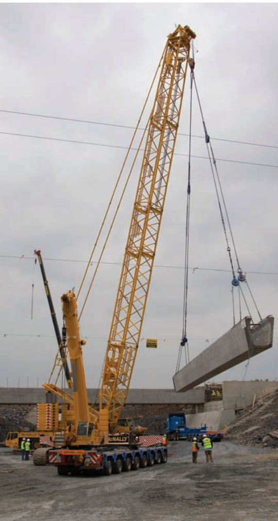
← Figure 7 Erecting a concrete beam (Southern Ring Road, Limerick, Ireland)
