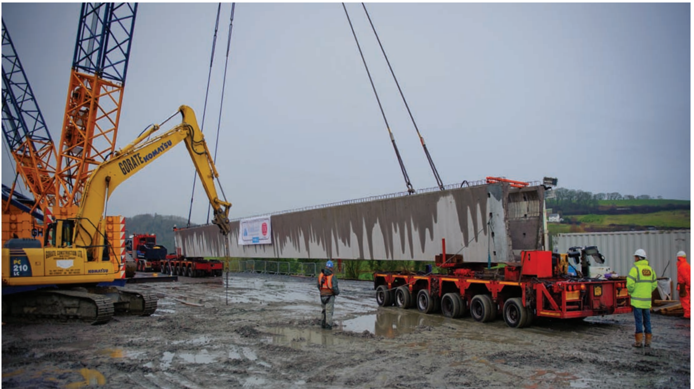
Figure 6 Transporting a concrete beam (Afon Hydfron Bridge, UK)
