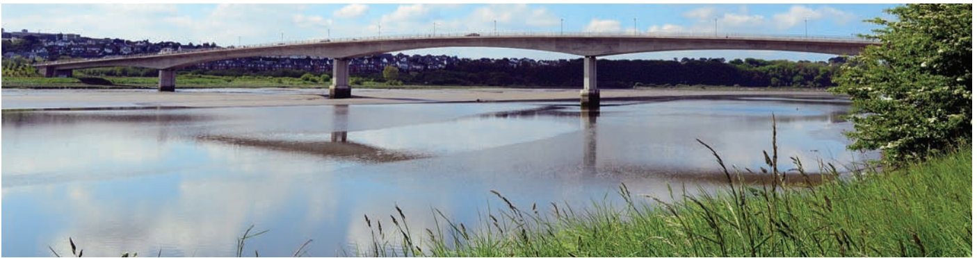
Figure 6 River Taw Bridge, Devon, UK
