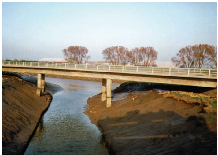
Figure 4 South Holland Bridge, Lincolnshire, UK
