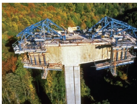
Figure 8 River Dee Viaduct, UK: balanced cantilever pair
