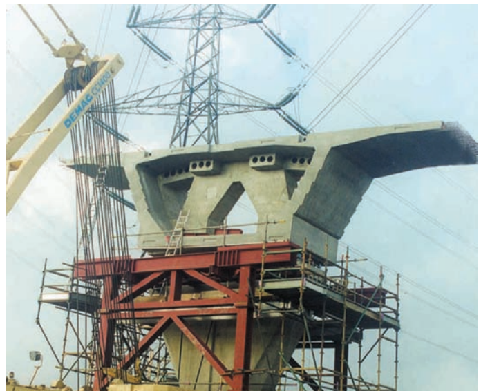
Figure 6 Crane-erected pier segment: A13 Viaduct, UK
