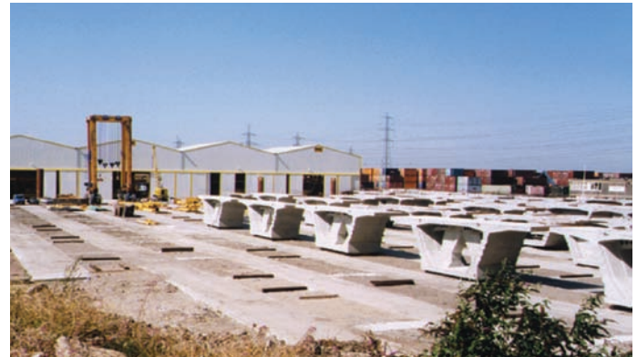
Figure 5 Segments in storage: A13 Viaduct, UK
