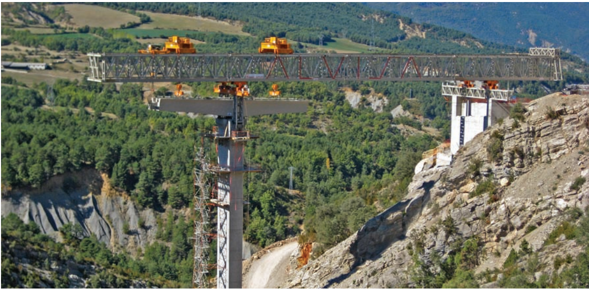
Figure 4 Egea Bridge, Spain: gantry-erected bespoke beams
