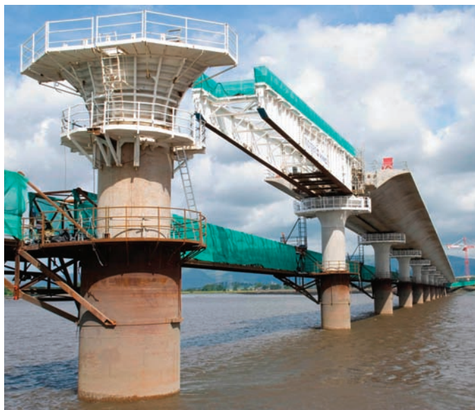
Figure 7 Launching nose: Clackmannanshire Bridge, UK
