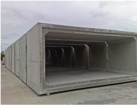
Figure 7 Standard precast culvert units
