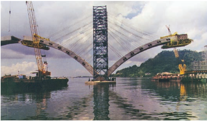
Figure 5 Sungai Dinding Bridge, Malaysia: balanced cantilever erection
