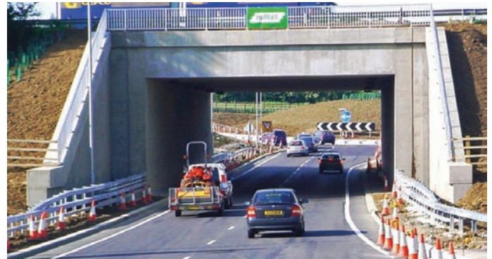
➔ Figure 10 Completed jacked box: A43 Bridge (under the M1), Northamptonshire, UK
