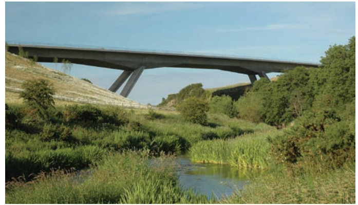
Figure 6 Framed legs: River Tyne Bridge, UK
