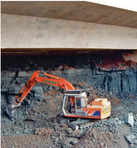
➔ Figure 10 Completed jacked box: A43 Bridge (under the M1), Northamptonshire, UK
