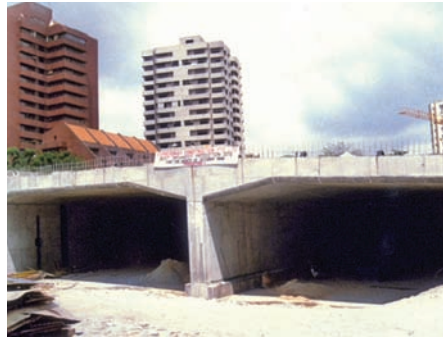
Figure 8 Singapore Central Expressway: 'bottom-up' construction
